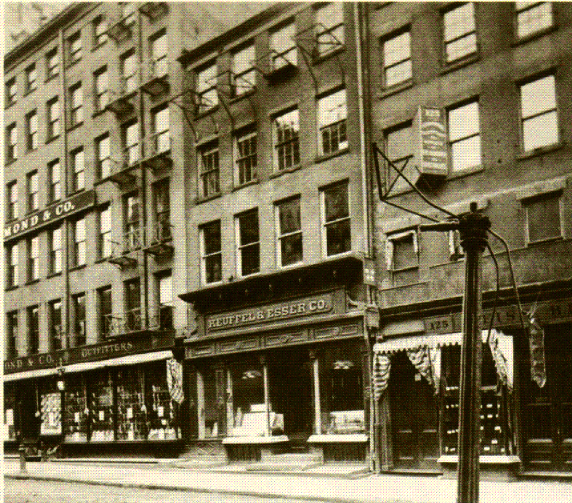
The first building at 127 Fulton Street, with blueprint racks showing on the fourth floor.
